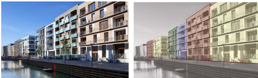
Figure 6.4: Establish 'fine grain' vertical and horizontal articulation (rhythm and scale) Sluseholmen, Copenhagen, Denmark
